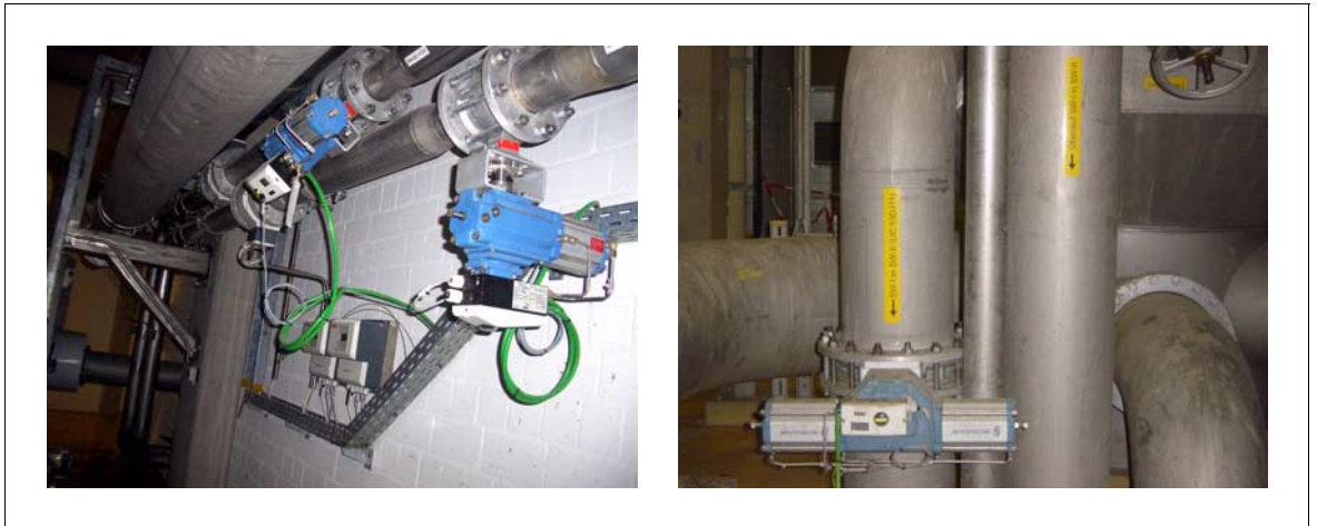
Fig. 5-1: Control valves in approach-flow system
