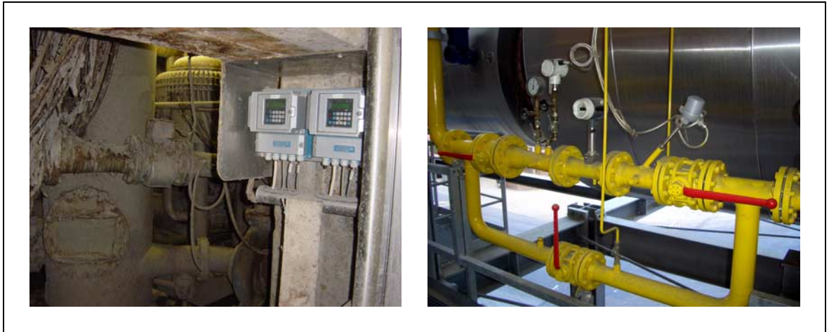
Fig. 2-1: Flow measurement at the KM 3
