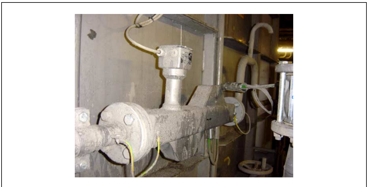
Fig. 4-1: Massflow measurement in white water 1
