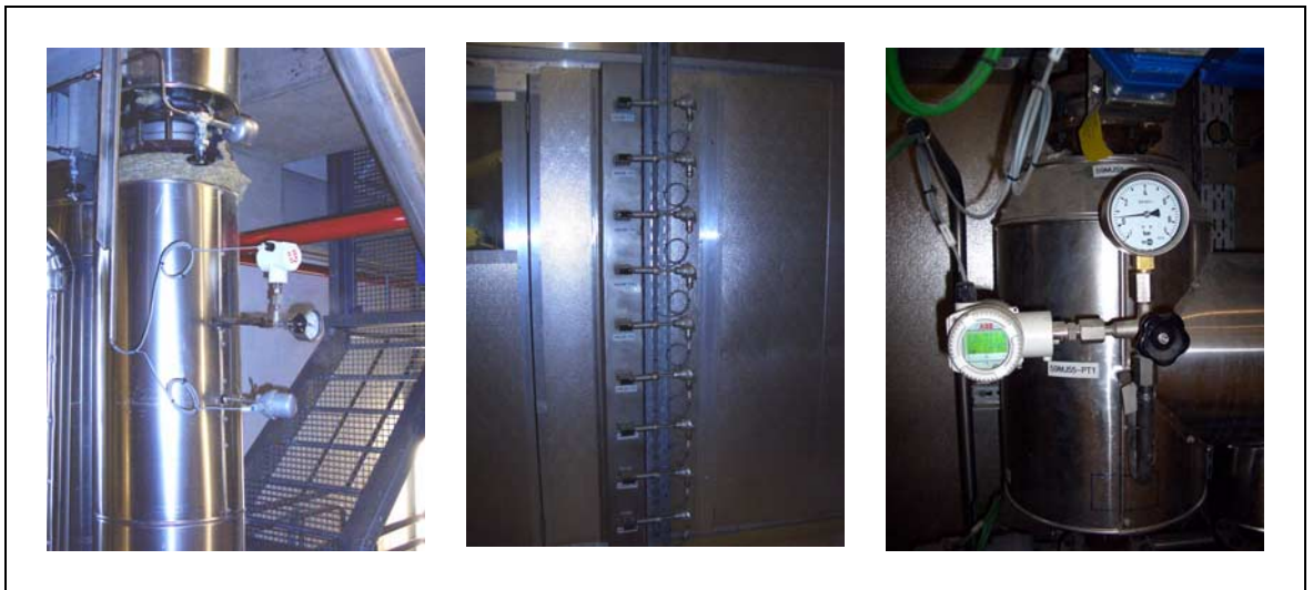
Fig. 6-1: Temperature and pressure measurement in steam and condensate systems
