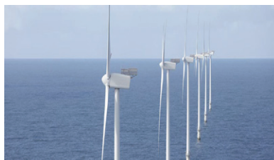
CGNPC Yangjiang Nanpeng Island Offshore Wind Power
