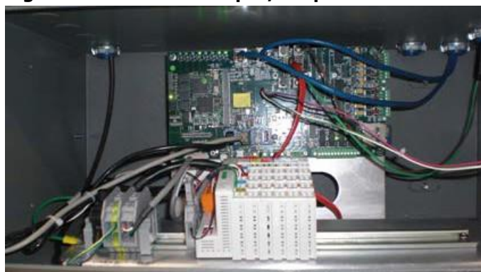
Figure 5-19: Internal Input/Output Module Locations
