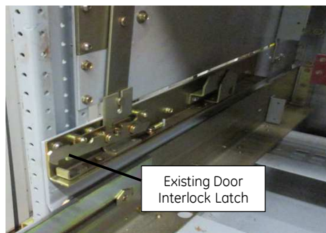
Figure 30B. AKD-10—Door Interlocking Components for WPS-32/WPH-32/WPX-32/WPS-40/ WPX-40/WPS-50/ WPX-50 Breaker.
