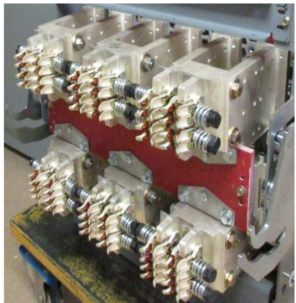
Figure 7A. AKD-10—Primary Contacts or “Fingers” (Apply Grease)
