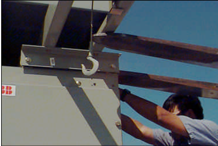
Figure 12. Push the Overhead Lift Device onto the rails.
