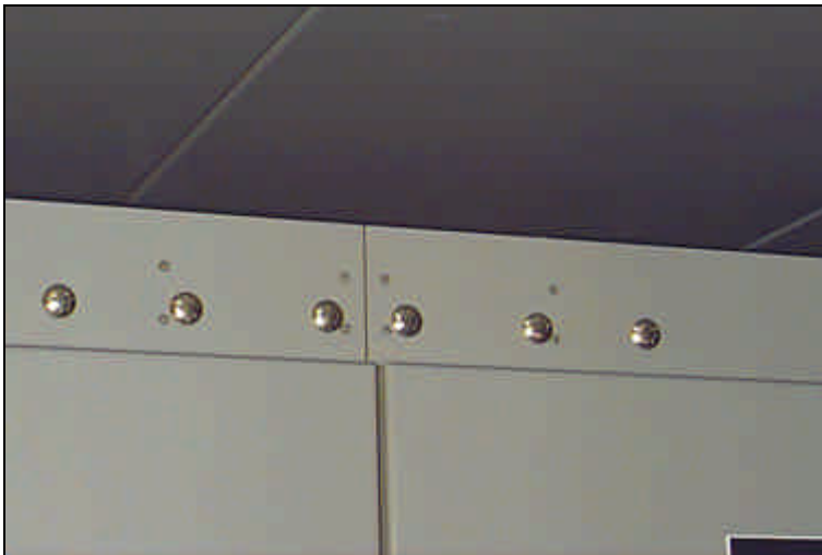
Figure 9. Secure plates and rails for a smooth and continuous transition between sections.
