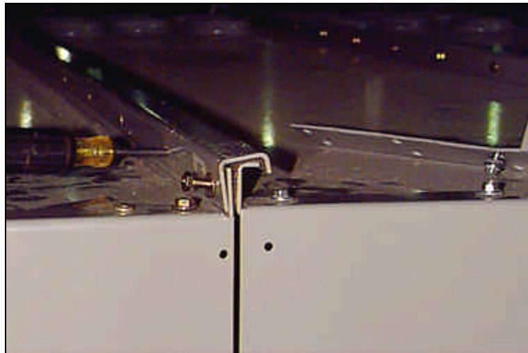
Figure 17. Loosely install the shipping split angle as shown.
