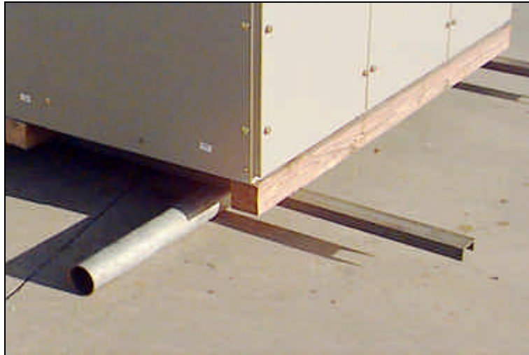
Figure 3. Position rails on rollers as shown for lateral moving.
