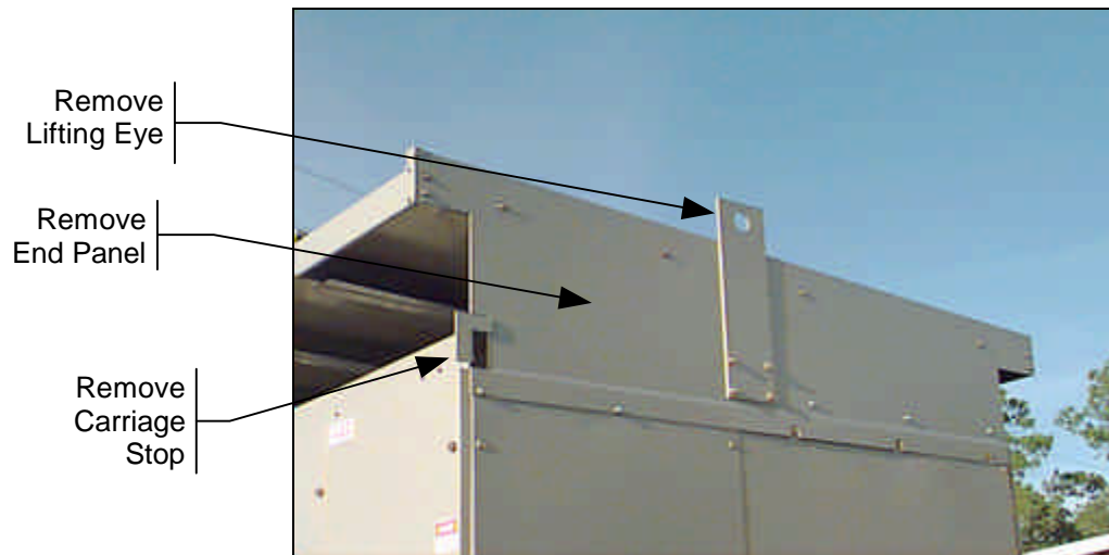
Figure 7. Remove the Lifting Eye, Carriage Stop and End Panel.
