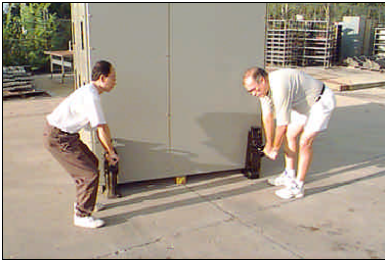
Figure 1. Position jacks under the front and rear corners, inside the shipping base.
