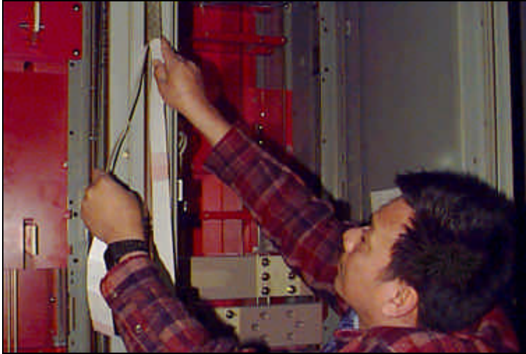
Figure 14. Install gasket material between shipping splits before bolting together.
