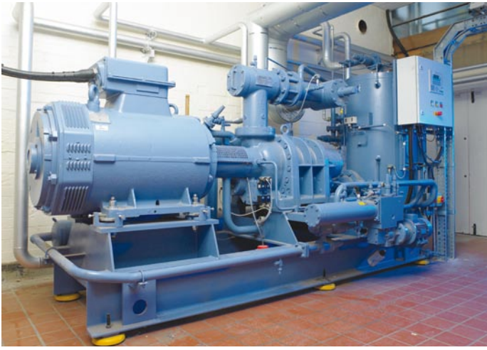
The compressor uses a low harmonic, ABB industrial drive.
