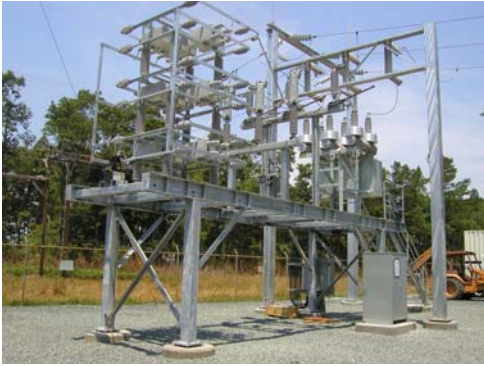
Picture shows 69kV Modular Capacitor Bank and Circuit Breaker.
