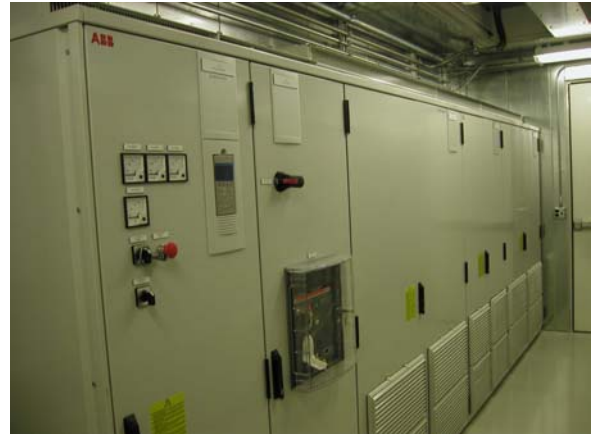
Picture shows inverter modules in one section of building.
