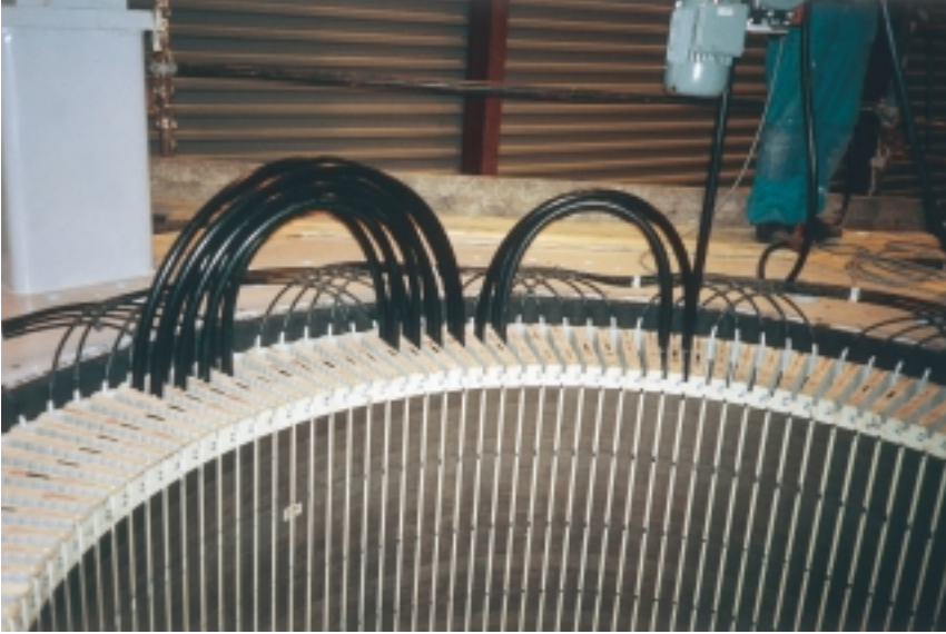
Porjus stator under construction. Here, the cable is being threaded through the bores.
