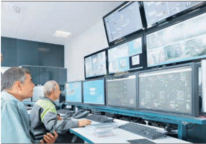
ABB's Extended Automation System 800xA controls the entire plant and each piece of equipment throughout the mine.
