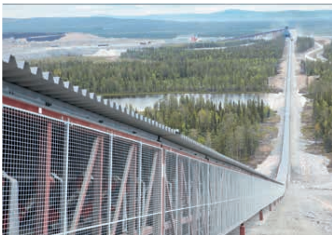
4 ABB drives are installed in the 7 km of conveyors that transport the ore to the concentrator plant at Aitik.
