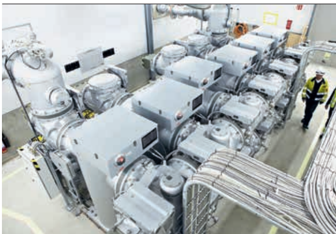
5 ABB's 170 kV gas-insulated switchgear distributes electric power to the mine.
