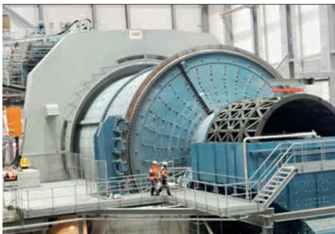
6 ABB's gearless mill drives power two massive grinding mills, which are the world's largest at 13.7 m long and 11.6 m in diameter.
