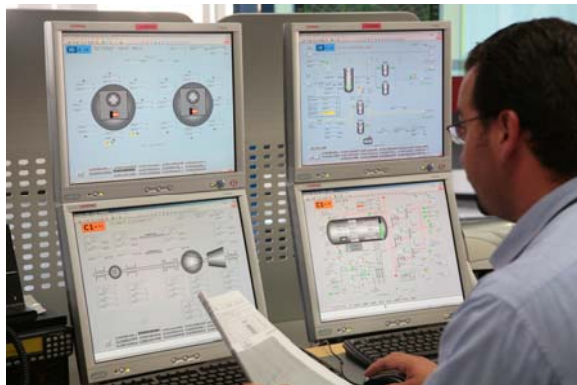
Figure 4 - Example of PGP graphics (Ferrera Erbognone, Italy, courtesy of Enipower, SpA)
