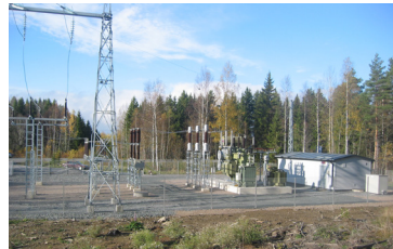
Distribution substations With 100 years experience, the world leader in turnkey air and gas insulated substations
