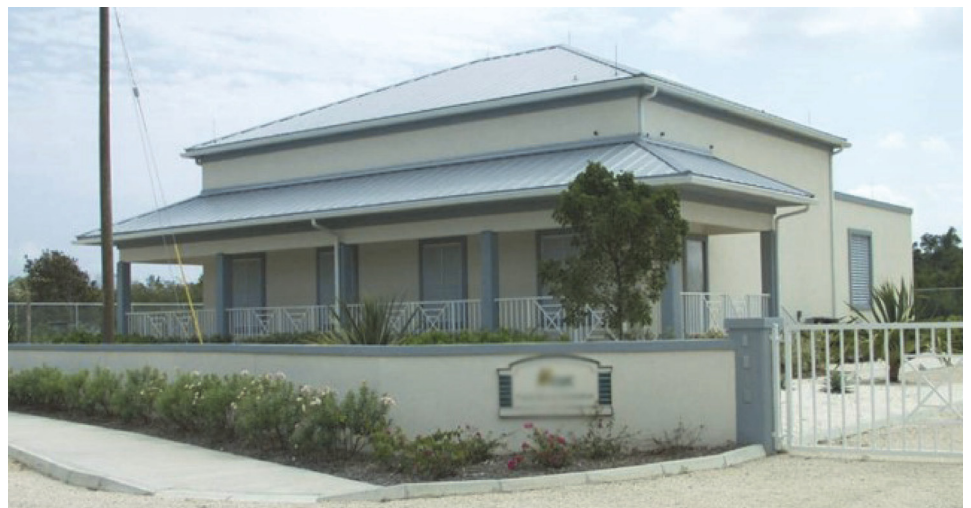
Indoor GIS substations blend architecture into the surrounding area for camouflage.
