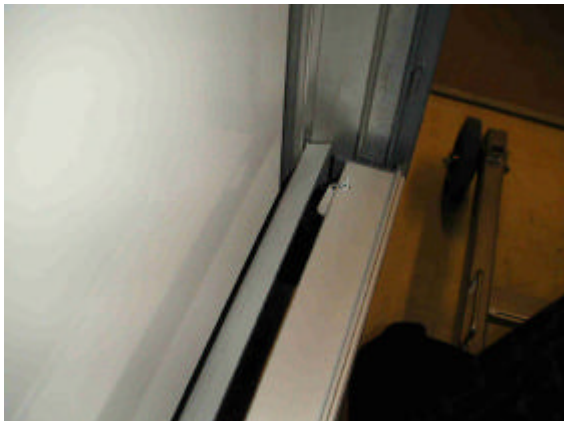
3.3 Remove the locking clip so the door falls down.
