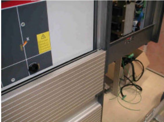
3.1 Dismantling the door.
