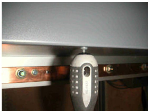
6.18 Mount the plastic rivet.
