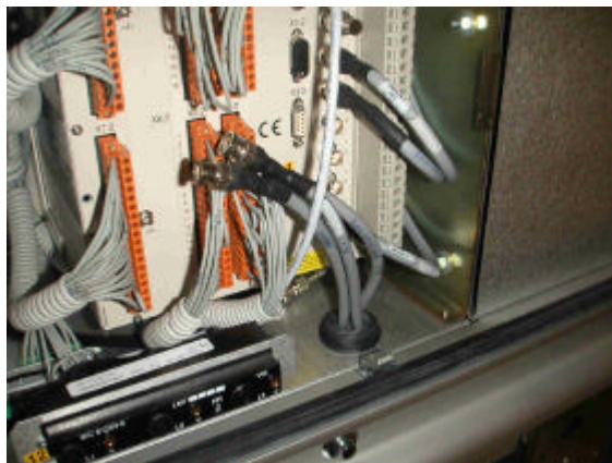
6.16 If the circuit breaker have current measuring you have to connect the sensor cables to the REF.
