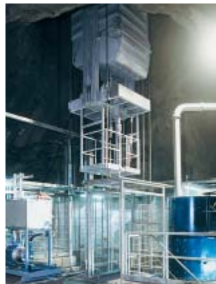
Skip with lower inspection platform
