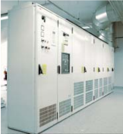
ACS600 drive for the production hoist
