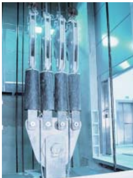
Rope attachments for the production hoist
