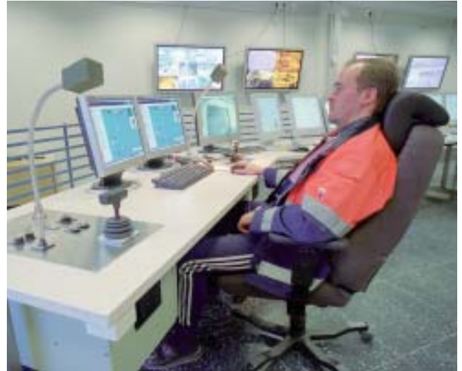
The central control room at Kemi Mine
