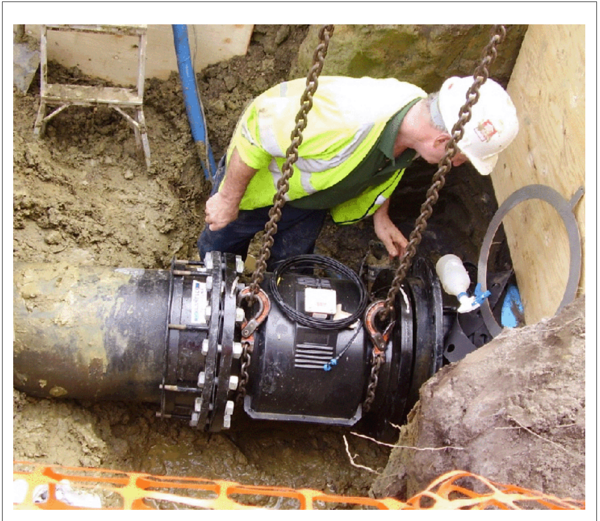
Fig. 2-5: Around 900 AquaMasters have already been installed throughout C2C's operating area, with more meters planned where additional flow data is required
