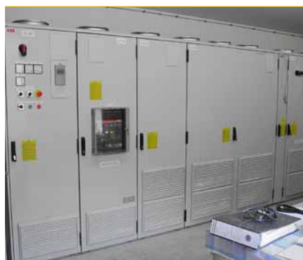
10 Multidrive panels for the downhill conveyor [2]
