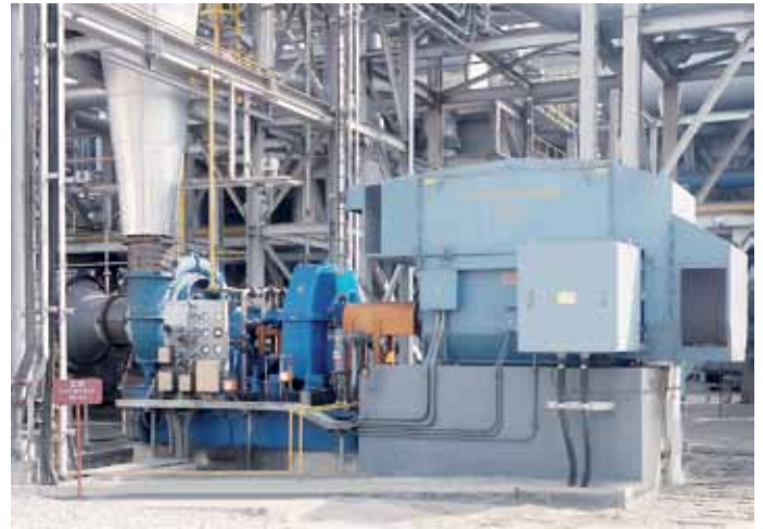
Pump motor soft started by the ACS5000 to reduce mechanical wear and tear.
