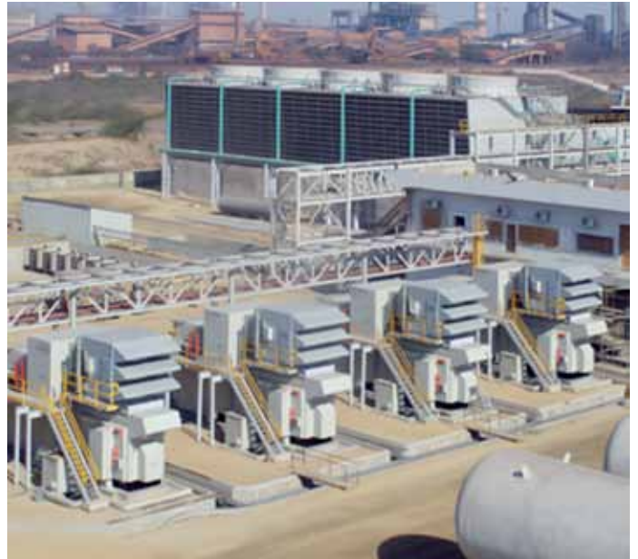
The Al-Tuwairqi Steel Mill Ltd in Pakistan.
