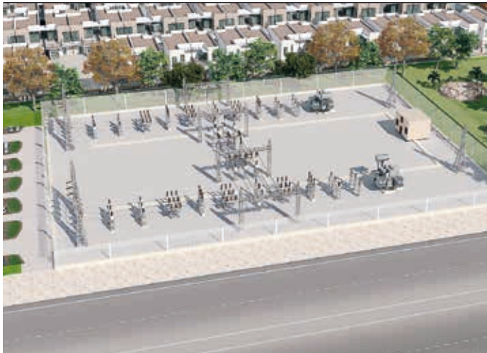
4a Air-insulated switchgear
