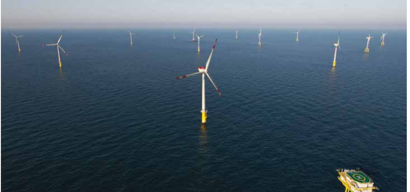
alpha ventus, also known as Borkum West I, Germany's first offshore wind farm (source: AREVA Wind, Jan Oelker)
