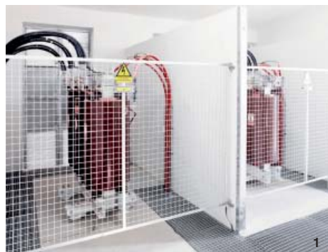
1 EcoDry in a substation | 2 EcoDry in industry | 3 EcoDry with renewable energies
