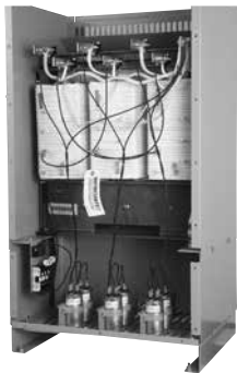
Guard II™ Transformer, (front panel removed)
