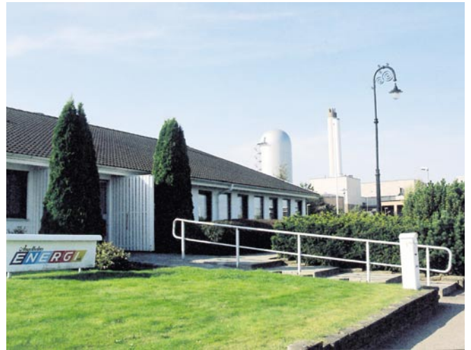
Ängelholm CHP plant in southern Sweden uses wood chips and natural gas as fuels.
