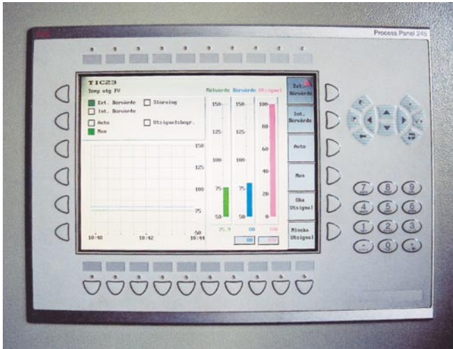
The Process Panel operator interface at one of back-up hot-water plants
