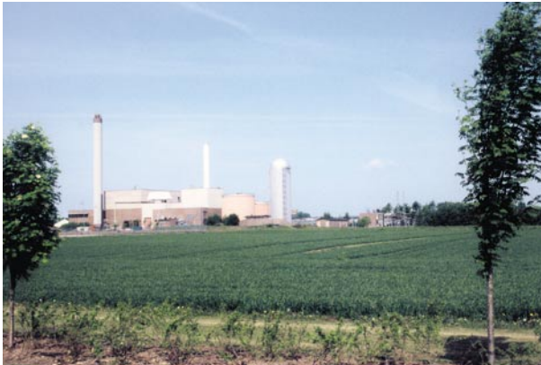
The Ängelholm CHP plant
