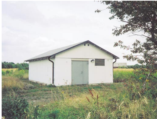
Pumpstation for the Luntertuns town district
