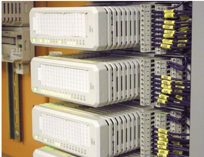
AC 800M controllers are using distributed I/O modules from the S 800I/O family for connection to the process
