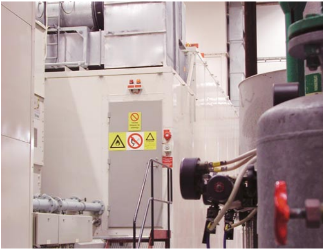
Interior from the Luntertun pump station
