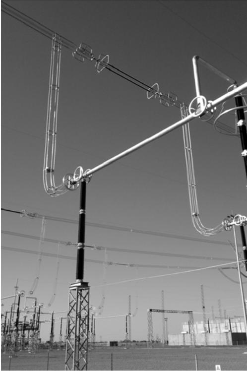
Fig. 6. Flying insulator and droppers for one Beta platform.
