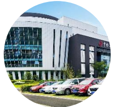
7 Kunshan Jinqiao Data Center China
