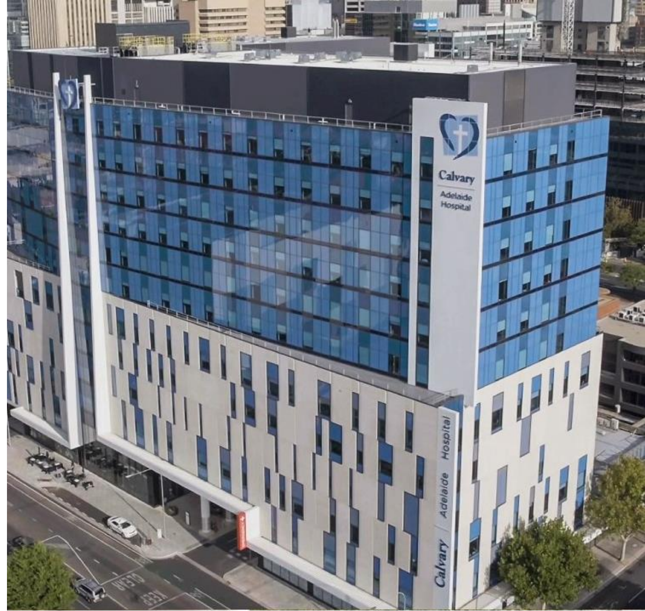
Calvary Adelaide Hospital, Australia Solution: Building Automation solutions
