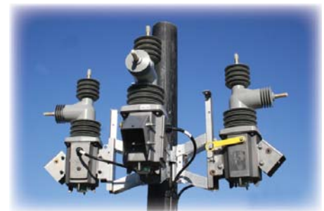
The OVR-3SP adds the functionality of three individually housed poles.
