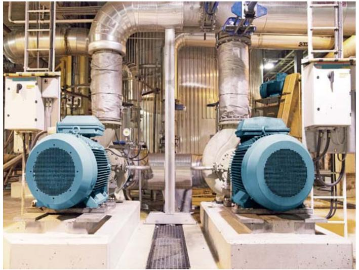
The energy comparisons were made using the new IE4 synchronous reluctance motor (left) and an older ABB motor (right).
