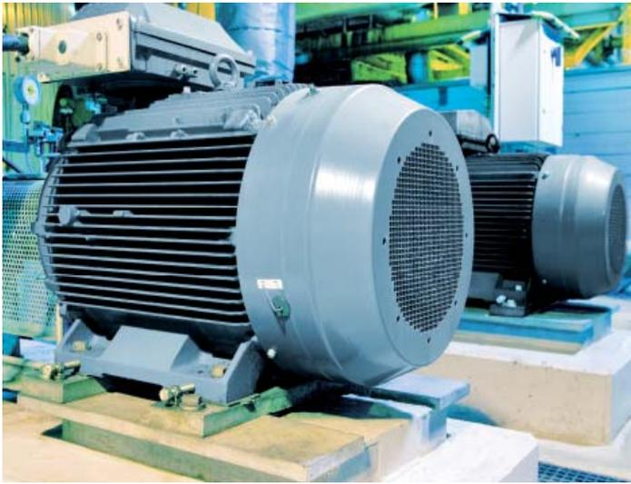
Looks the same. The new IE4 synchronous reluctance motor (foreground) has the same footprint and frame size as the older ABB motor it replaced.
