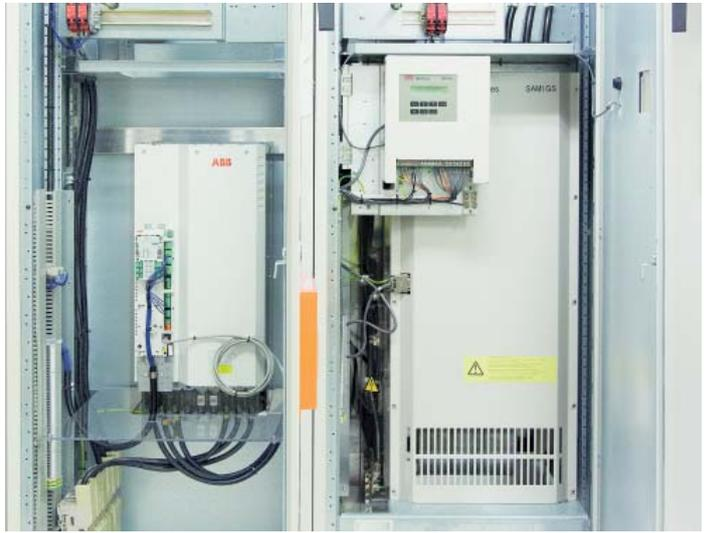
The new ACS850 variable speed drive (left) replaced an older ABB Sami GS drive, similar to the one on the right.
