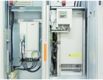
The new ACS850 variable speed drive (left) replaced an older ABB Sami GS drive, similar to the one on the right.
