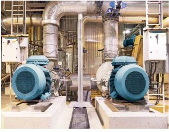
The energy comparisons were made using the new IE4 synchronous reluctance motor (left) and an older ABB motor (right).
