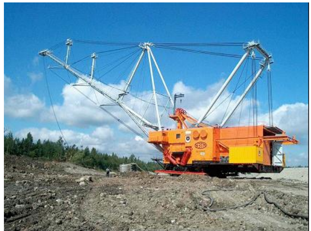
Figure 2: Modernization of the Mechanical and Electrical equipment of the Dragline Type 15/90 in Estonia, 2005
