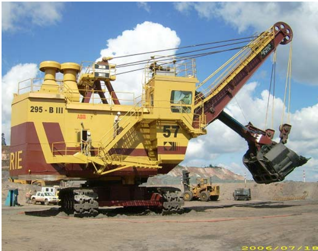
Figure 3: Refit of the Shovel BE295 BIII with ABB AC Drives for Mining in Brazil, 2006
