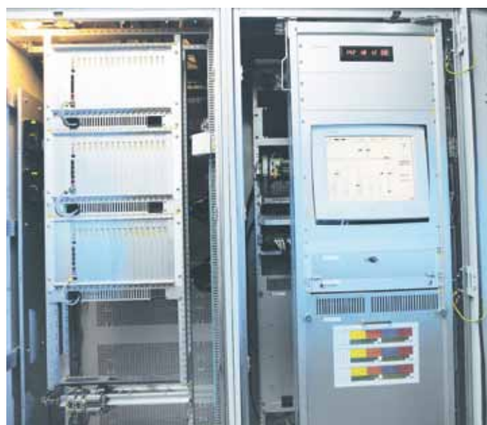
MACH 2 constituents: Valve Control Unit and HMI.
