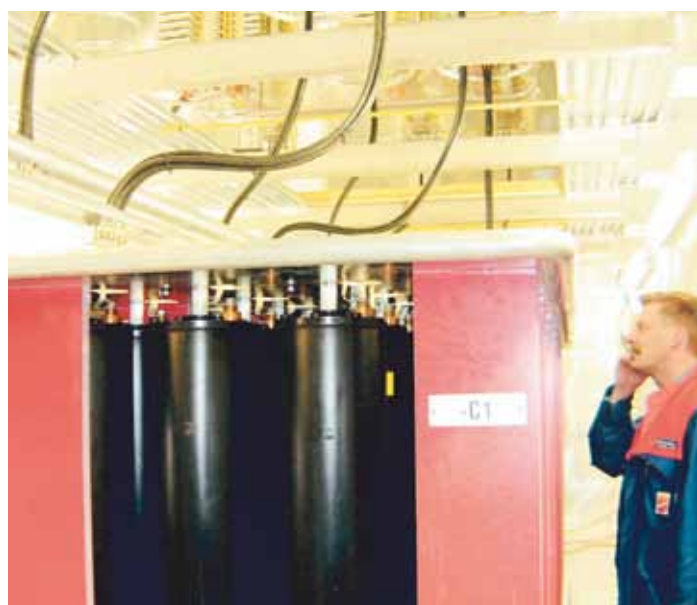
Dry-type DC capacitors for SVC Light®.
