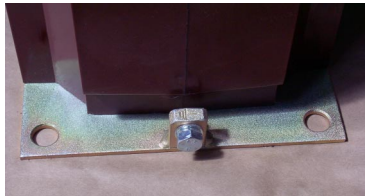
Figure 14. Location of fixing holes behind VT
