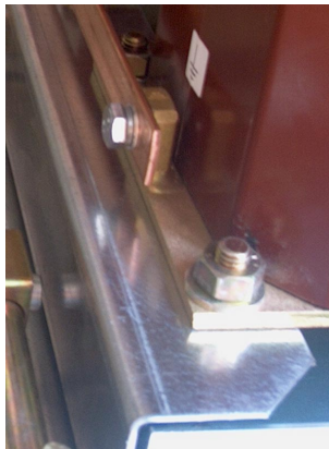
Figure 16. Fixing bolt behind VT
