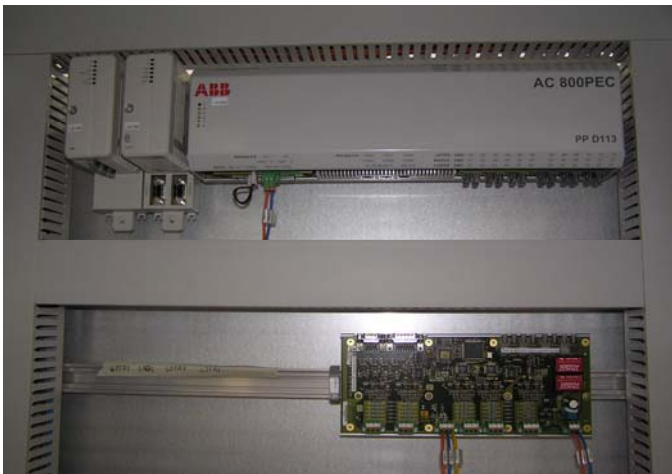
Figure 6. New drive controller built into cycloconverter.
