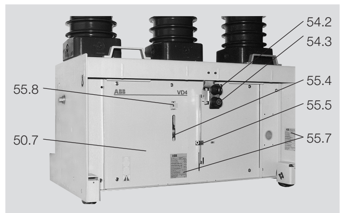
Figure 3/4: Indicators and control on a circuit-breaker for fixed installation
