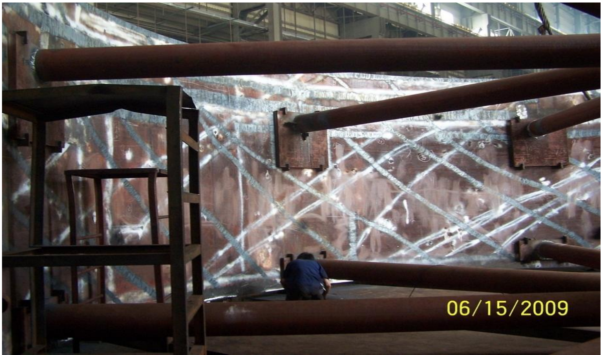
Figure 3 – Uncontrolled heat straightening
