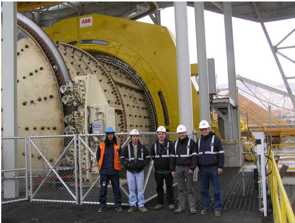
Figure 8 – Yanacocha gearless motor
