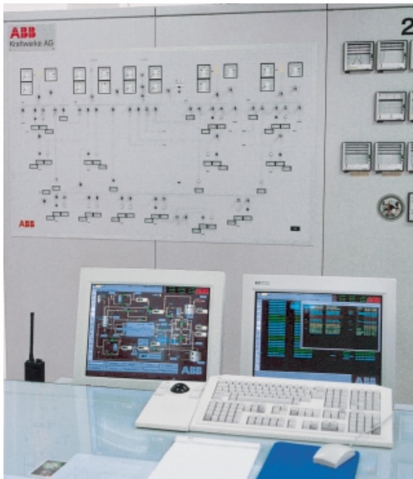
Operator station in the central control room
