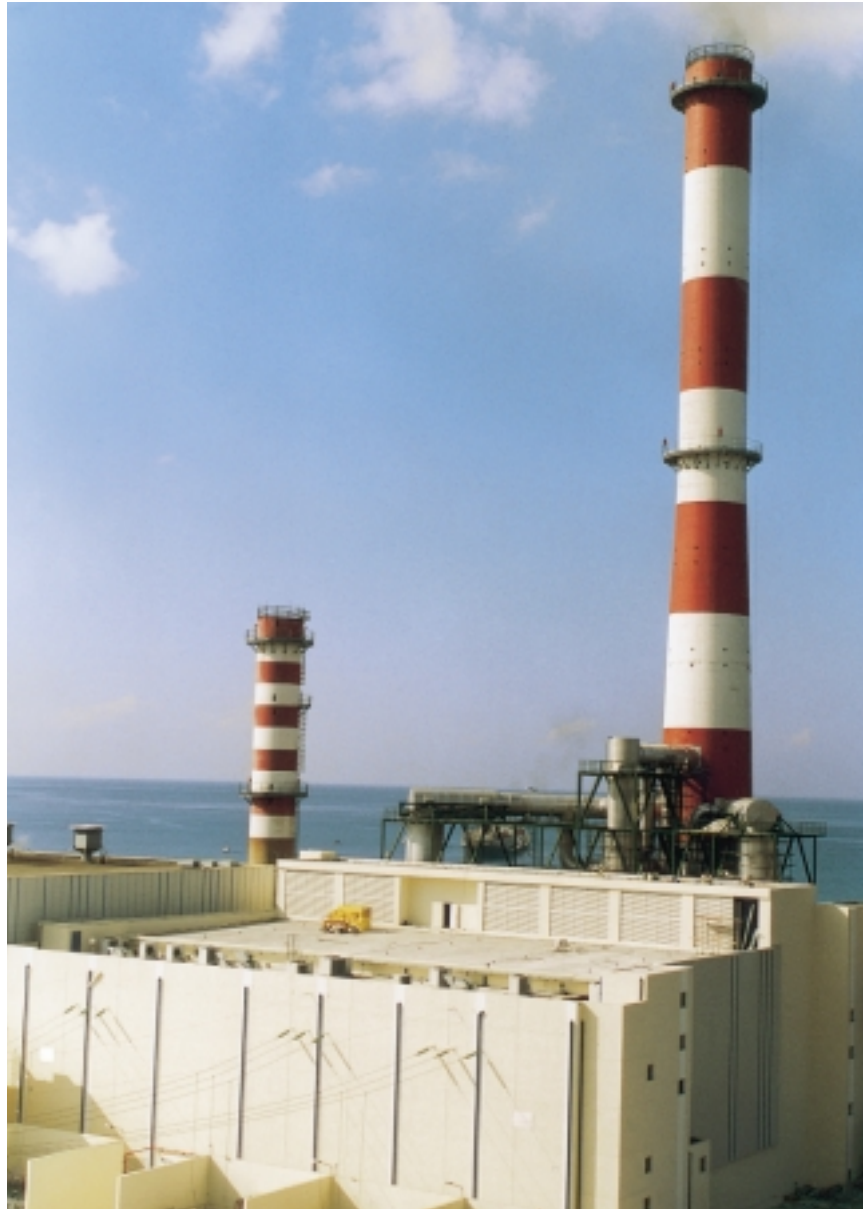
Rhodes diesel power plant, today with two 12-MW and three 24-MW units 1
