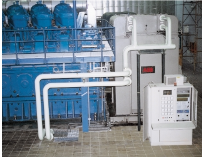
One of the three 24-MW diesel-generator sets
