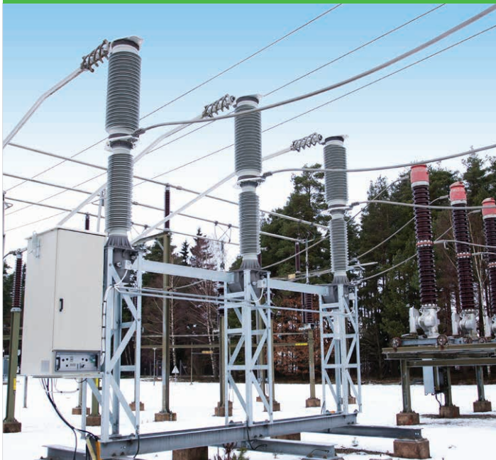
Pilot live tank breaker LTA, 145 kV in 2010
