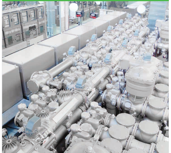
World's first eco-efficient GIS 170 kV in 2015
