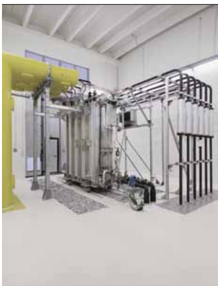
5 AC Excitation Transformer with the 3 bus ducts (yellow on the left) for primary windings supply and the 6 bus connection to the 12 pulse ARU
