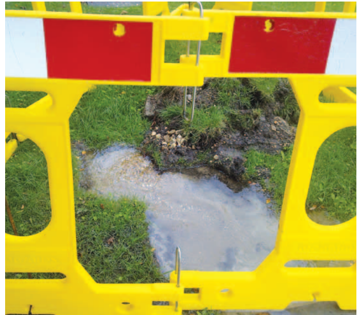
Losses stemming from small but steady leaks can be hard to detect.
