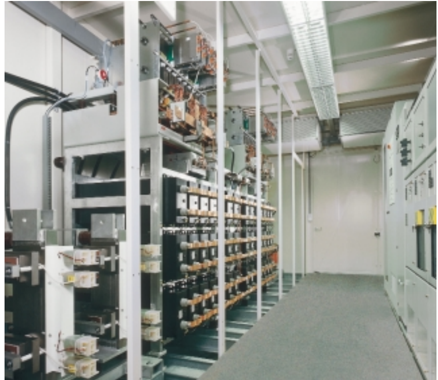
DC capacitors, IGCT converter module and electronic short-circuit device of the Dynamic Voltage Restorer 11
