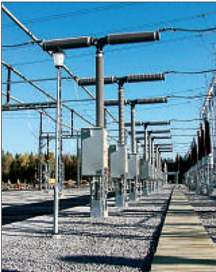
oil hydraulic power circuit breaker drives. As this technology is now outdated compared with current state-of-the-art designs, relatively intense servicing is required to keep them operating satisfactorily.
