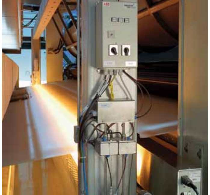
Example of an operating area next to a hazard area
