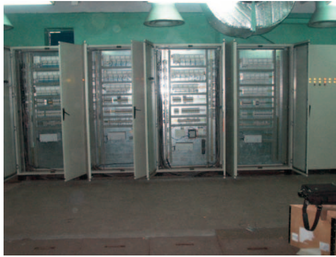
Electrical Room with ABB's Control System.
