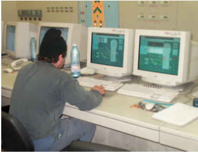
Two Operate™ Process Portal workplaces in the control room.
