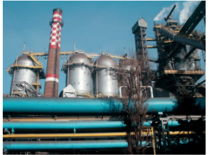
General view of BF#1 after its modernization.
