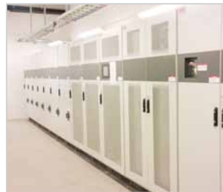
Final installation of the PCS100 UPS-I system
