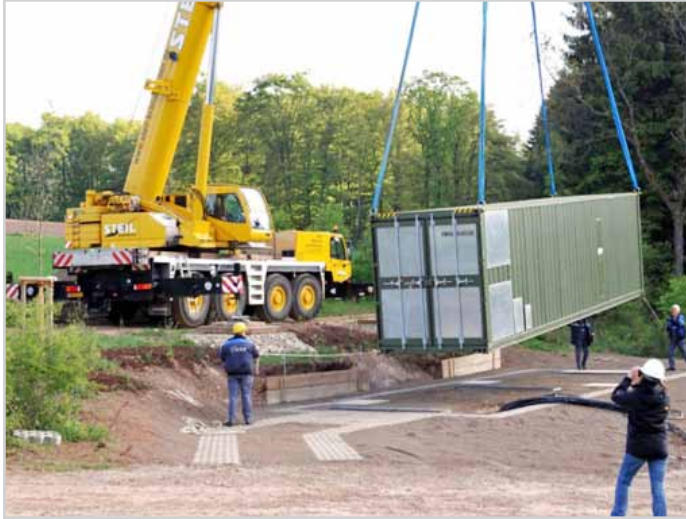
A heavy-duty crane positions the medium-voltage regulator onto its base with care and absolute precision (photo: RWE).
