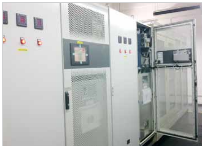
The 175 kVA AVCs are protecting the fiber production lines
