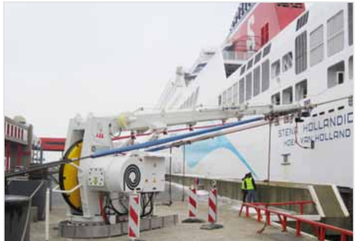
Connecting Stena Hollandica to the local grid
