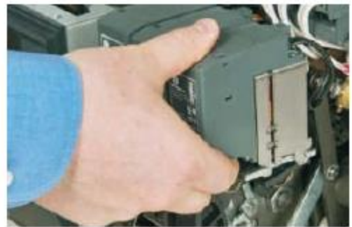
Figure 4. Shunt Trip Assembly
