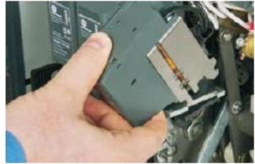
Figure 3. Shunt Trip Inserting
