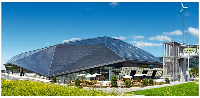
Thanks to innovative technologies, ABB has reduced the energy consumption of Umwelt Arena Switzerland by 30%. So for example, the PMA® conduits are used in the building-integrated photovoltaic installation to protect DC power cables.
