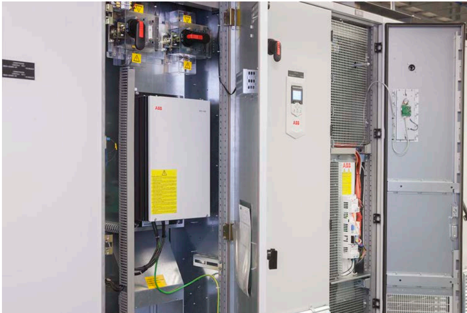
Old drive (left) and retrofitted drive (right)
