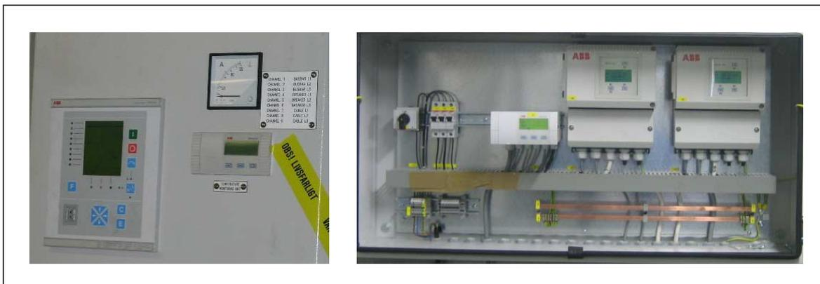
Fig. 3-1: FCU400-P flow computer unit as a field-mounting device placed on Z rails in a switch cabinet (right-hand side) or as a panel-mounting device integrated in the switch cabinet front door (left-hand side)
