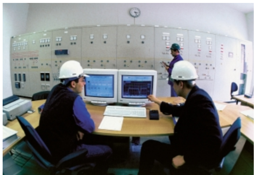
Control room with mimic diagram. In the foreground are the MMI monitors. 7
