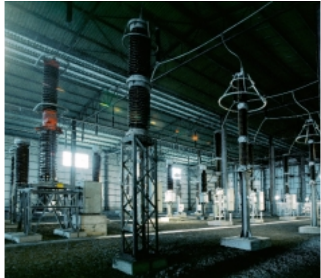
220-kV indoor switchyard of ISAL's Straumsvik smelter
