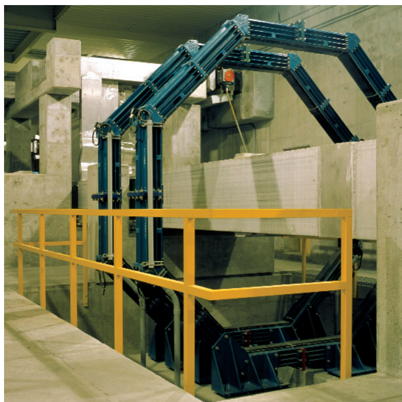
Fig. 2: Hall effect dc current transformers LEM LKP 400
