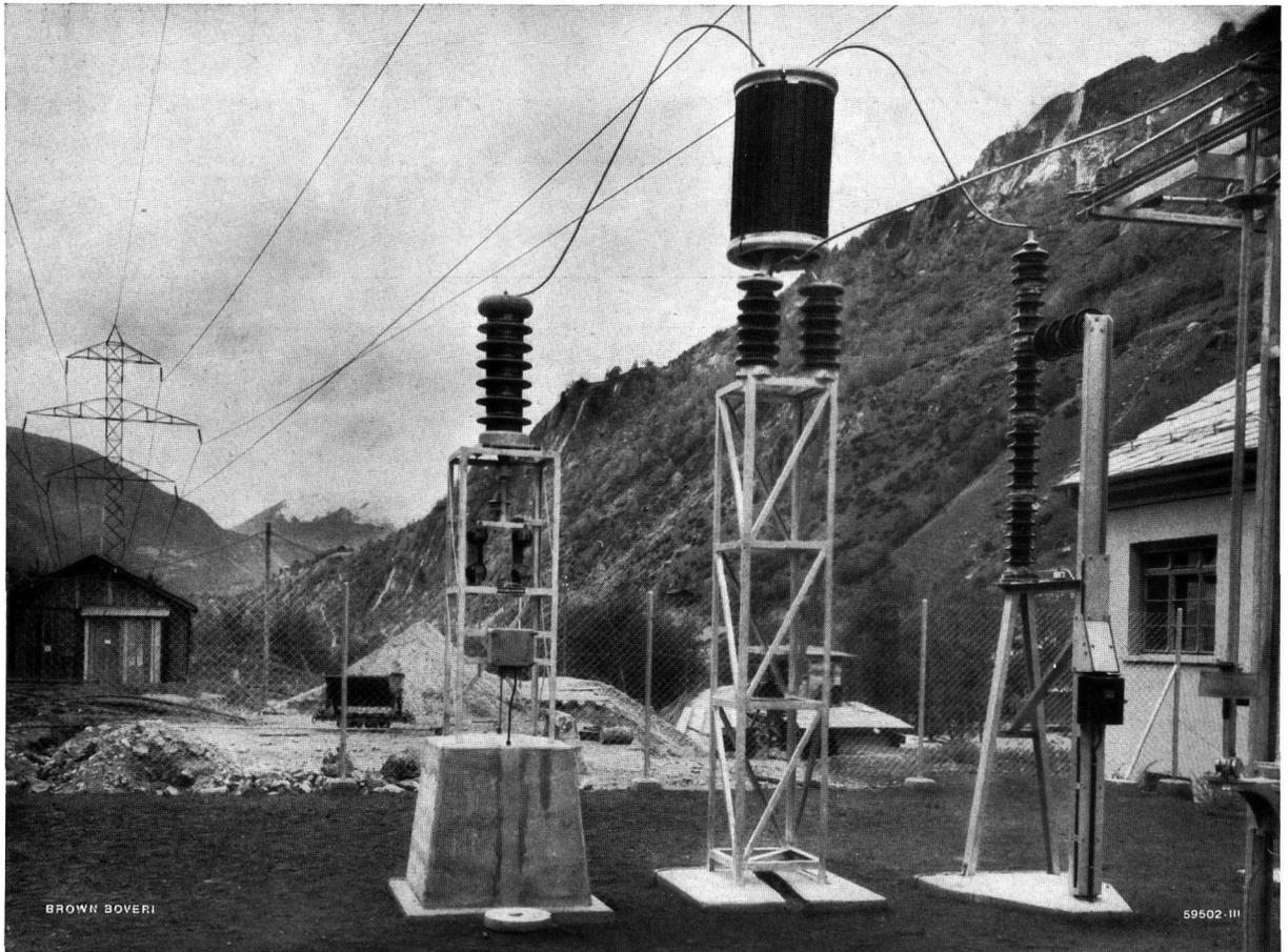
Coupling of a carrier-current telephony installation to a 65 kV line.
