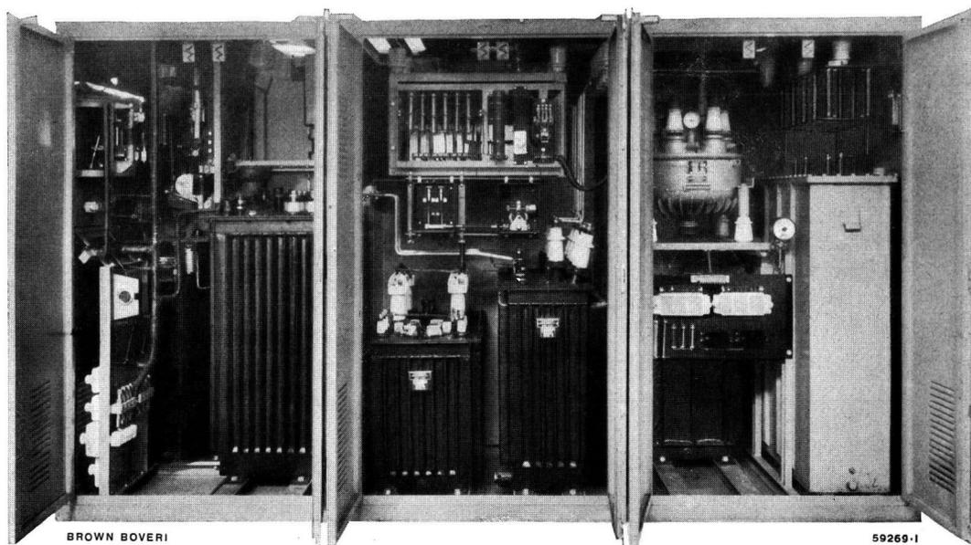
Fig. 3. — Transmitter power plant with associated high-voltage rectifier.
