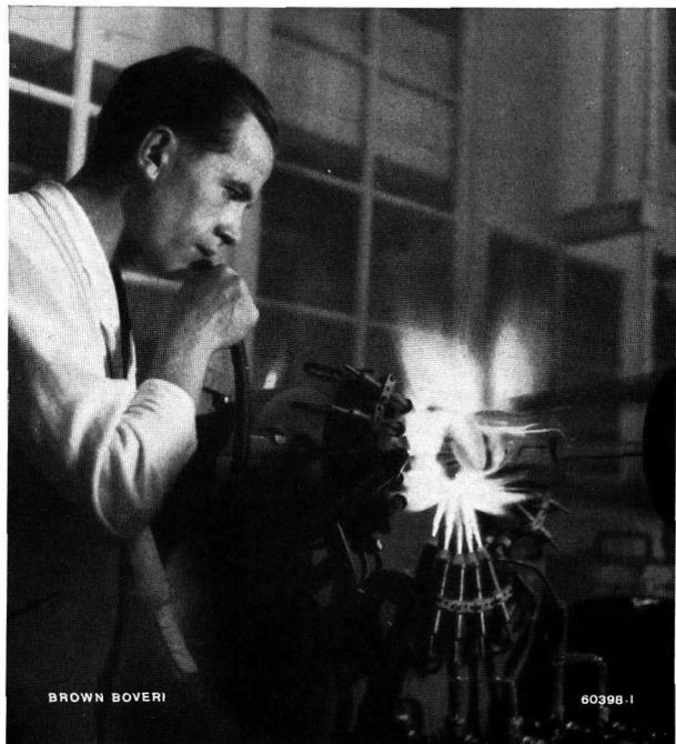
Fig. 1. — Glass lathe for fusing metal anodes to the glass envelopes of high-power transmitting tubes.
