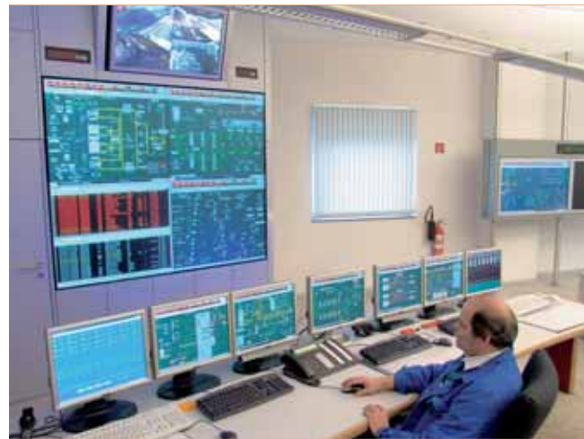
2 The new control room at Scholven
